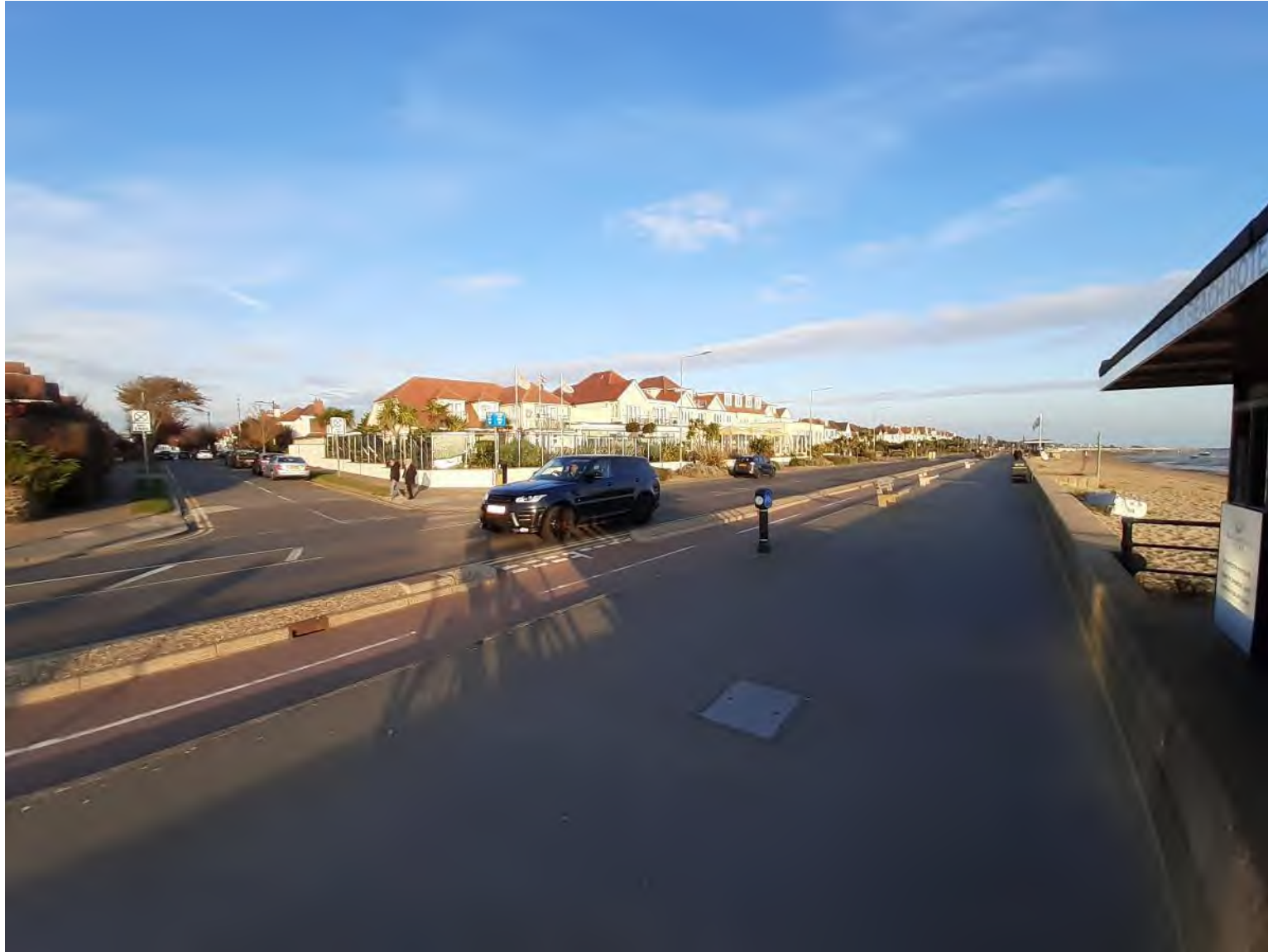
The site viewed from south-west
